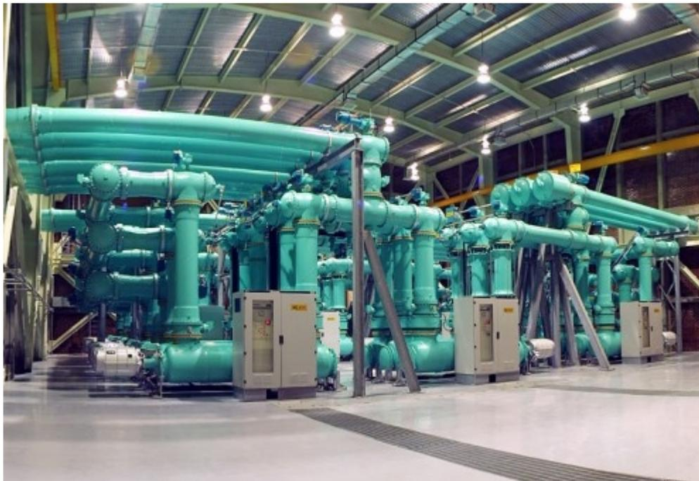
**Figure 4.2:** Gas insulated Substation
