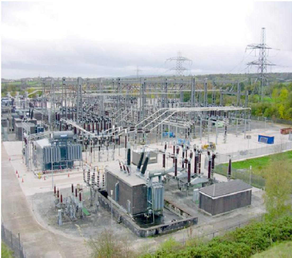
**Figure 4.3:** Air Insulated Substation (Source: <http://www.foxitsoftware.com>)
